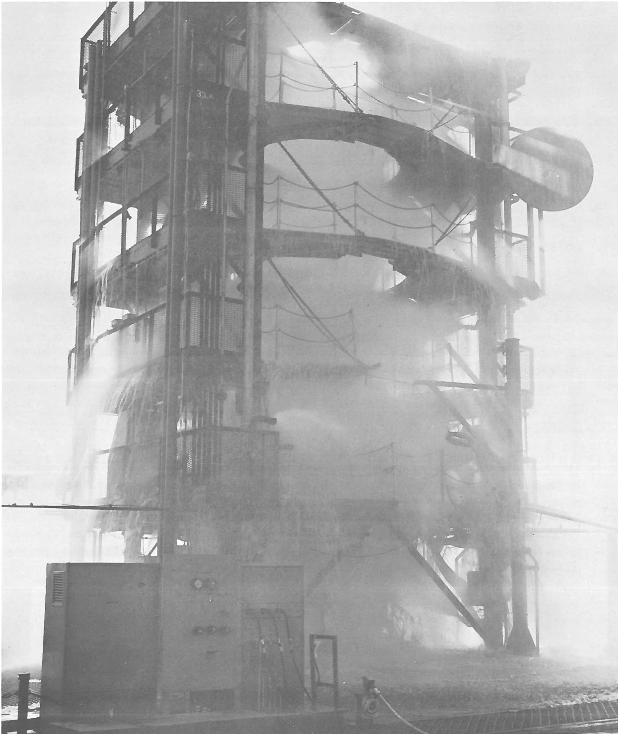
Figure 10. Water deluge system, Sycamore static test stand.
